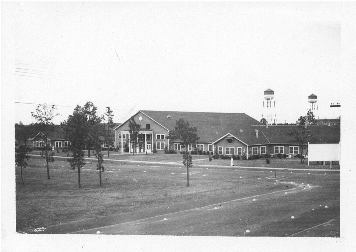
NAS PENSACOLA, FL. ADMINISTRATION BUILDING
